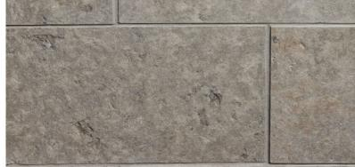
PANEL INSTALLATION SHOWN Mortar: Western Type- S Joint Type: raked Size-115/8" x 235/8" thermalled finish
